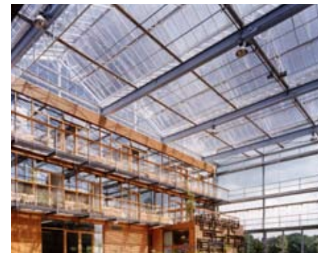
Above, a central atrium skylight illuminates the core of the administrative and community space level of the facility. This simple element reduces energy consumption while improving work conditions and the experience for visitors.
