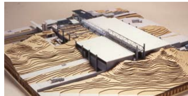
A model showing the use of desert berms to mitigate the scale of the facility. Soil fill used to raise the facility above flood levels was taken from the soil cut from the ground to create the retention pond. A balance of soil cut and fill is an important strategy to reduce pollution, costs, and energy.
