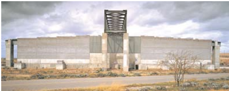
The giant truss structures create interior flexibility and allow for large sections of natural light to enter the building. Raw concrete was left untreated to blend more with the environment while reducing unnecessary cost and energy expenditures.
