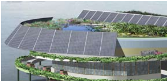
Left, south-facing photovoltaic panels and a central skylight reduce the facility's reliance on grid-supplied energy, potentially allowing the primary operations to function during a blackout.
