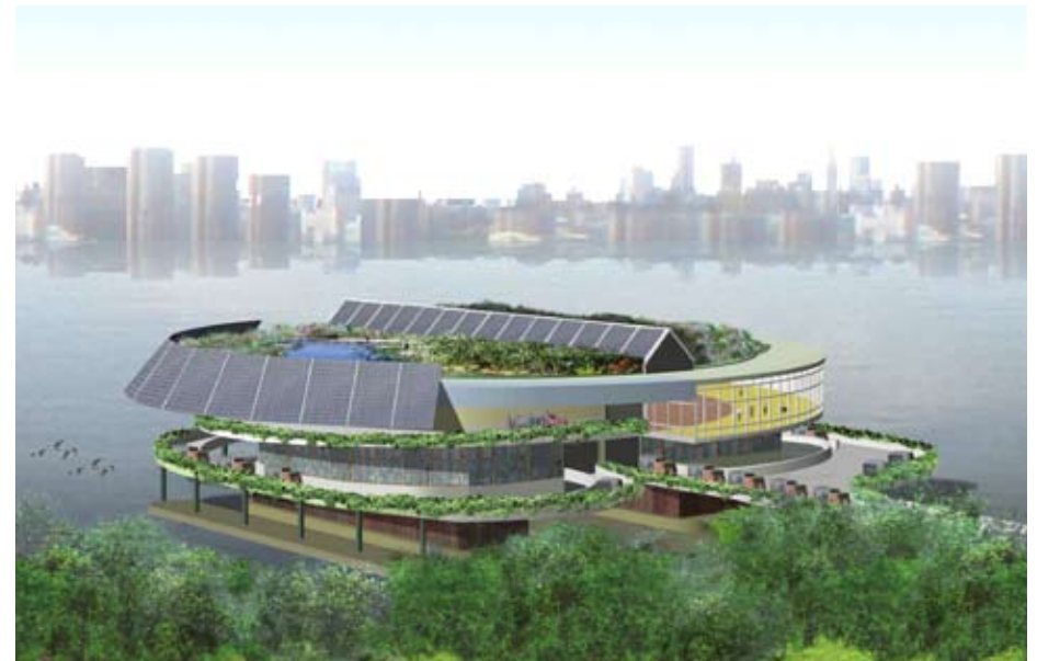
Above, a rendered view of the proposed Marine Transfer Station with a naturalized green roof, building-integrated solar panels, automated truck queuing ramps with vegetation buffers, and spaces for administration and public access.
