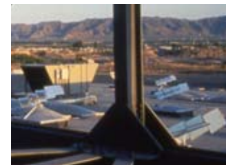
Left, heliostats (solar tracking mirrors) direct sunlight into the skylights at the Phoenix facility to increase natural light and reduce daytime peak energy consumption.
