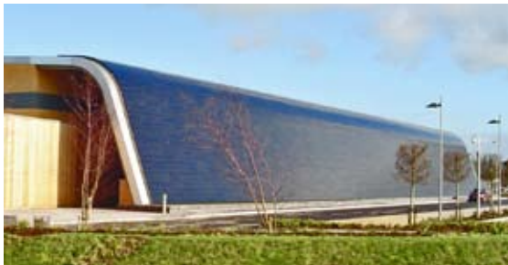
Left, an example of photovoltaic panels integrated into a building's facade. This system is a 85kW wall on the Welsh Development Agency Technology Center in St. Asaph, North Wales. The 11,000 square ft. solar wall produces energy equivalent to the needs of approximately 25 typical single family homes.
